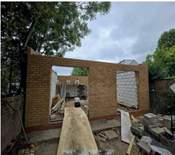
Stage 3: Brickwork (Wall)
